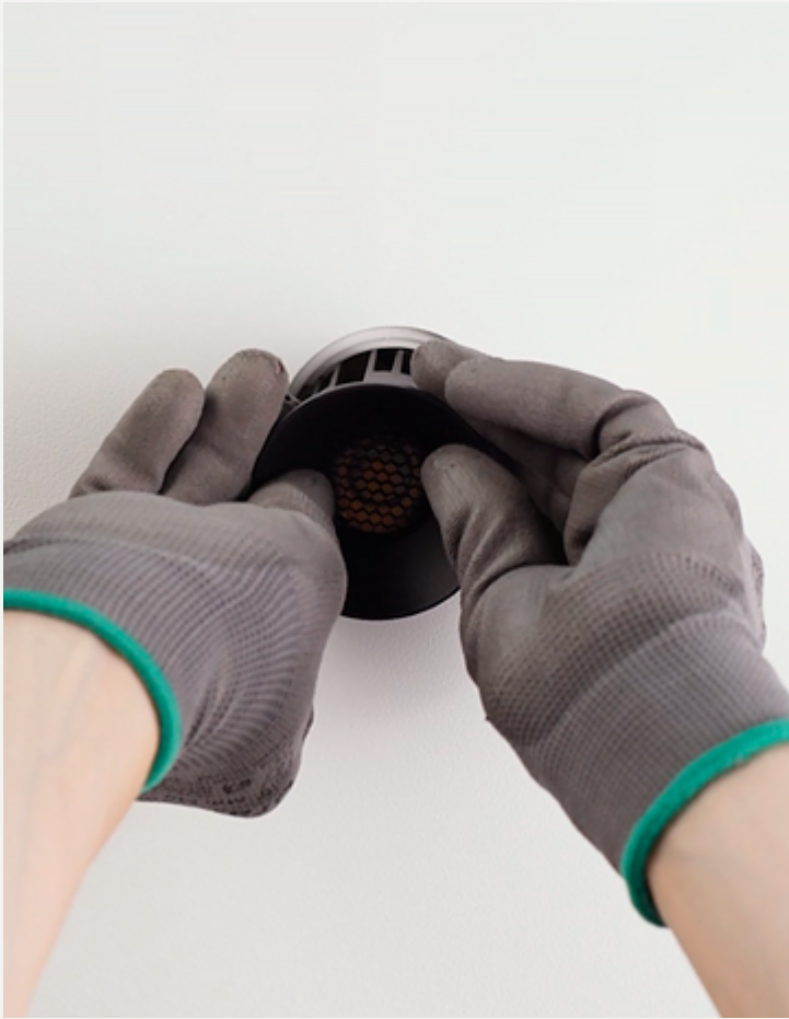
The luminaires can be leveled using the laser level, thanks to the special notches at 45° and 90°.
